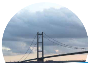
The Humber Bridge
