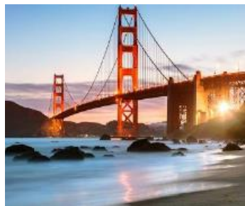
Golden Gate Bridge
