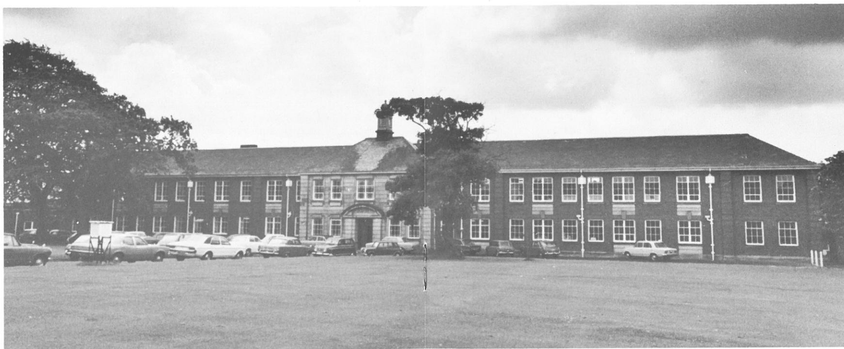
Church Road School 1931
