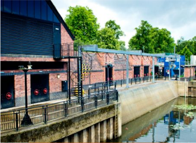
A flood defence wall
