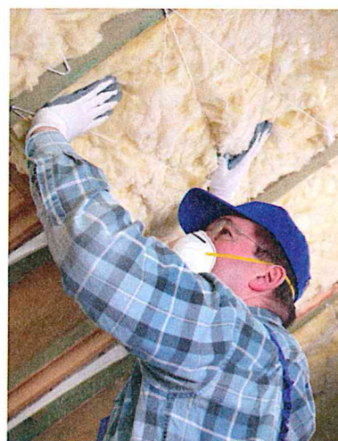
FIGURE 2.3.5c: Insulating a house.
