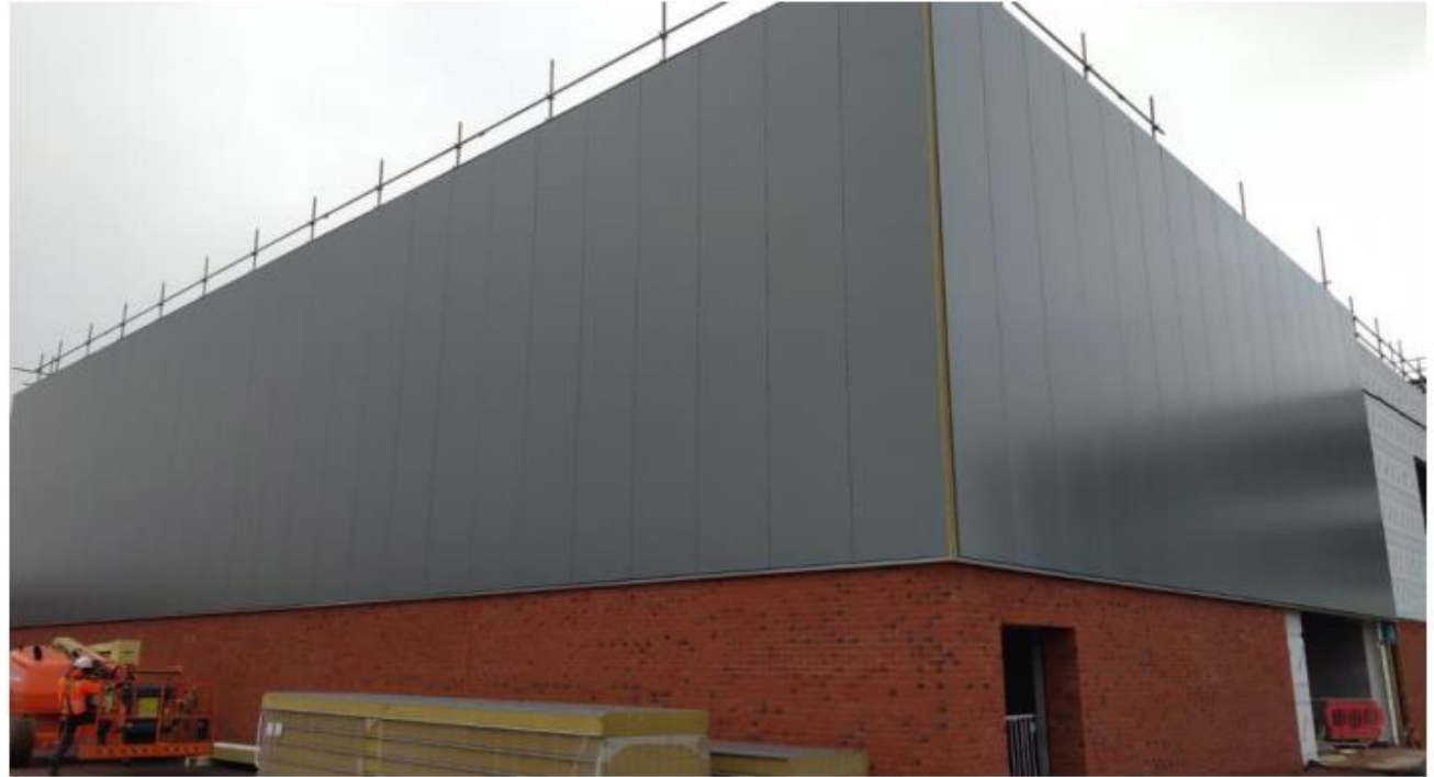
↑ Cladding to the sports hall installed as planned
