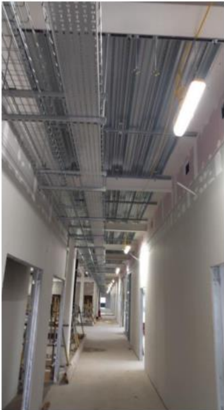
Electrical containment to first floor
