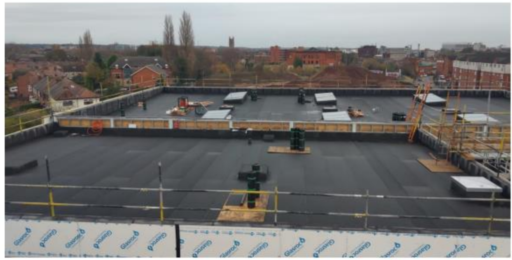
Roof complete to Sports, upstand links now underway ↑
