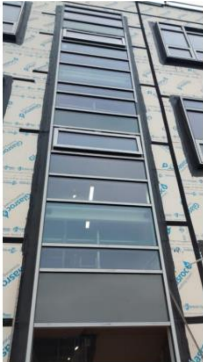
← Stairs Curtain walling glass now installed
