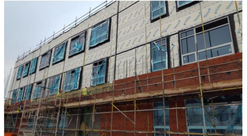
West elevation brickwork ongoing
