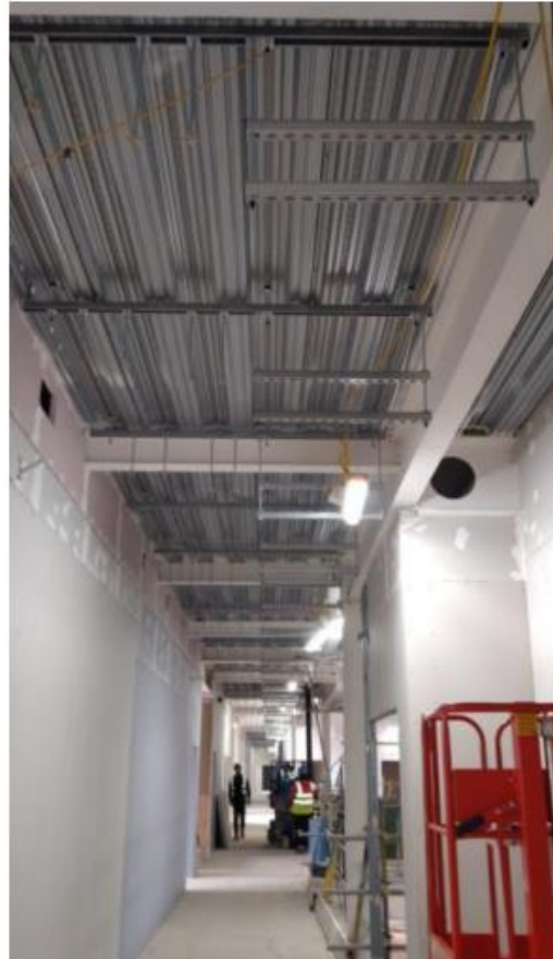
Electrical containment to first floor
