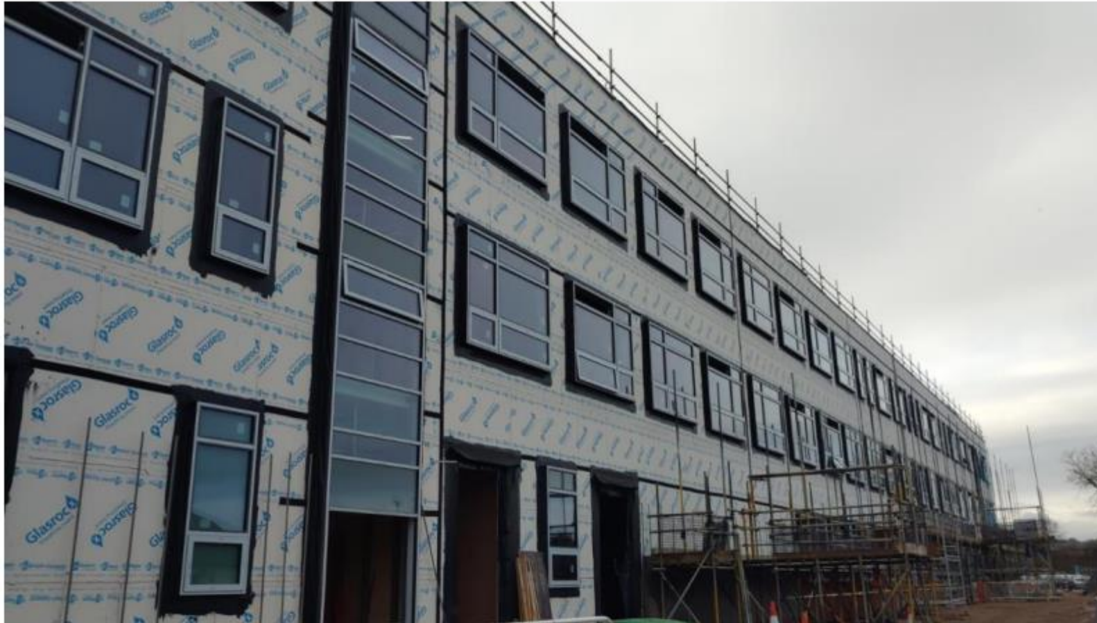
Northern elevation showing the completed window and curtain walling installations, note the brickwork creeping from the west.
