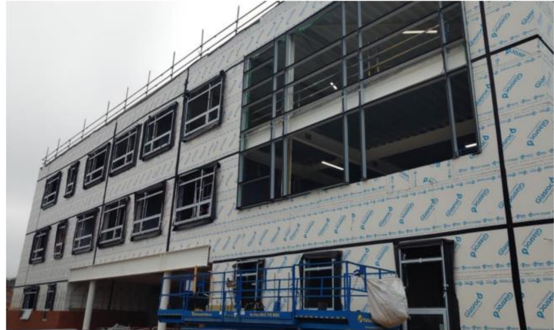
Eastern elevation with windows and curtain walling installed with glazing ongoing
