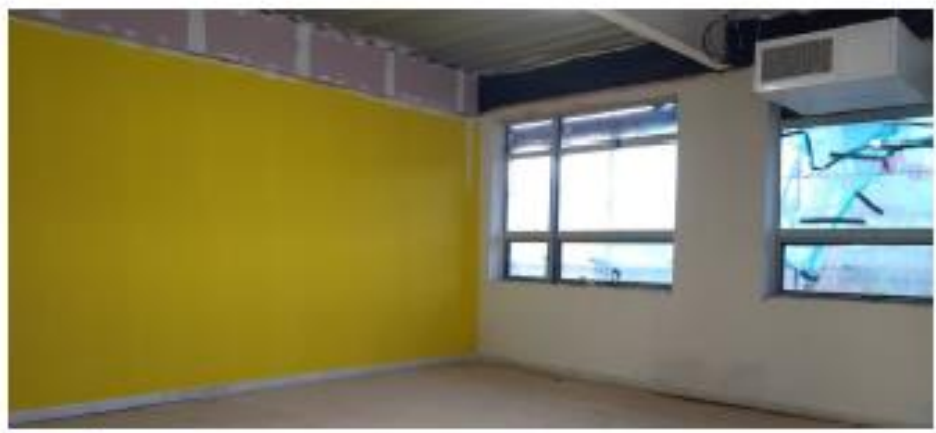
↑ Carpentry, decorations ? And NVHR install
