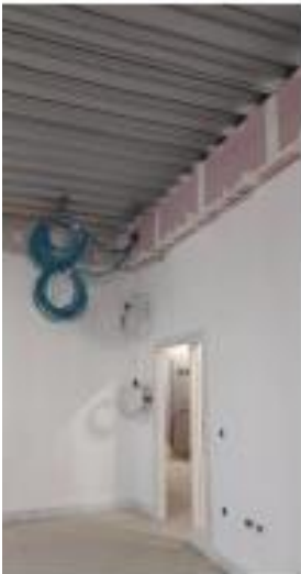
Feature walls and carpentry ongoing, data to rooms and NVHR wiring installed to classrooms
