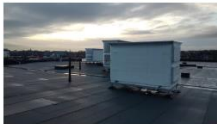
AHU's now installed to the roof with connection operations to commence in the next period.
