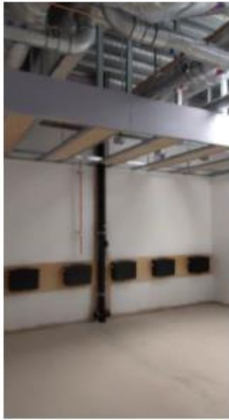
Toilets cisterns installed ready for flooring and IPS units
