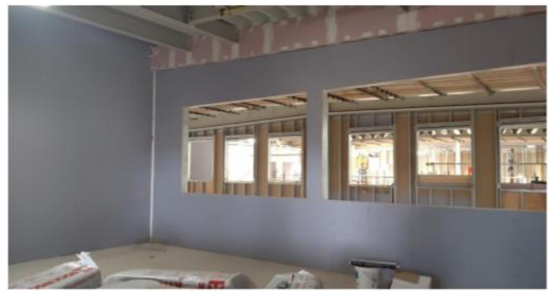
Boarding to atria windows ready for plaster
