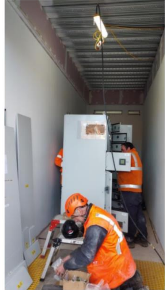
New Electric mains panel delivered and installed to the switch room
