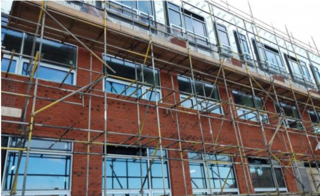
Brickwork to the north elevation now working on the second floor
