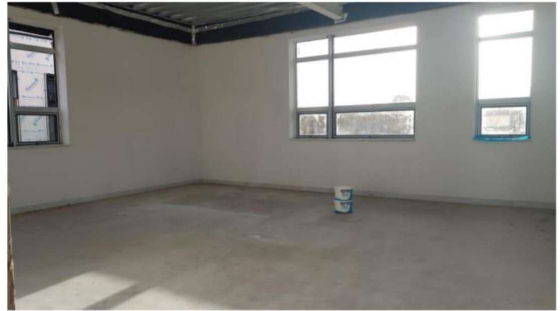
Plastering decoration and first fix joinery cills and skirtings
