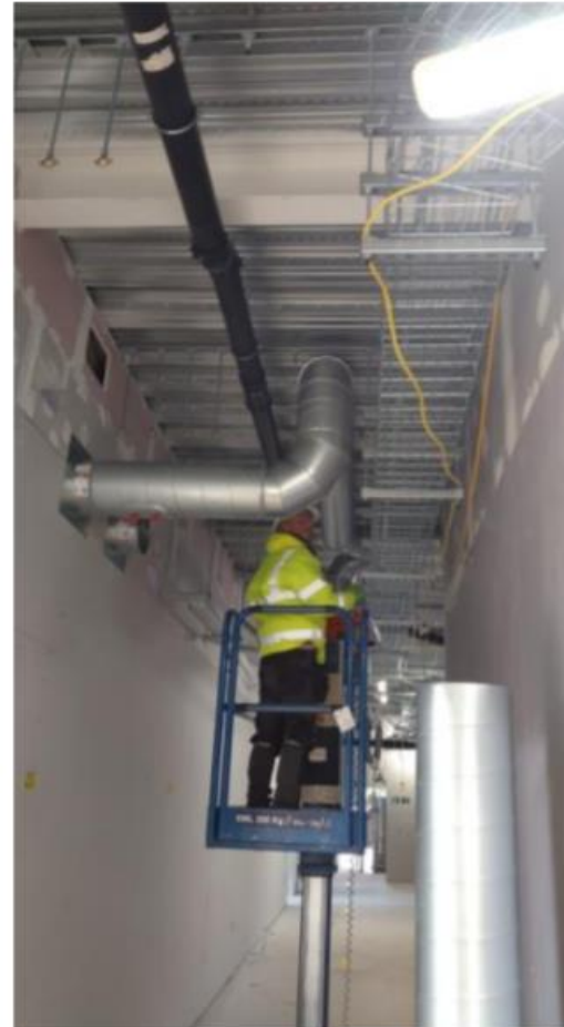
Duct work installations to ground floor
