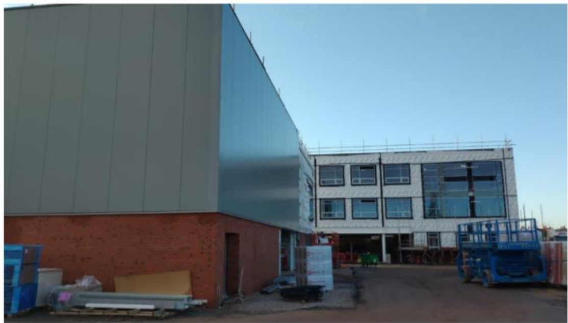
Undercroft Curtain walling and external brickwork ongoing
