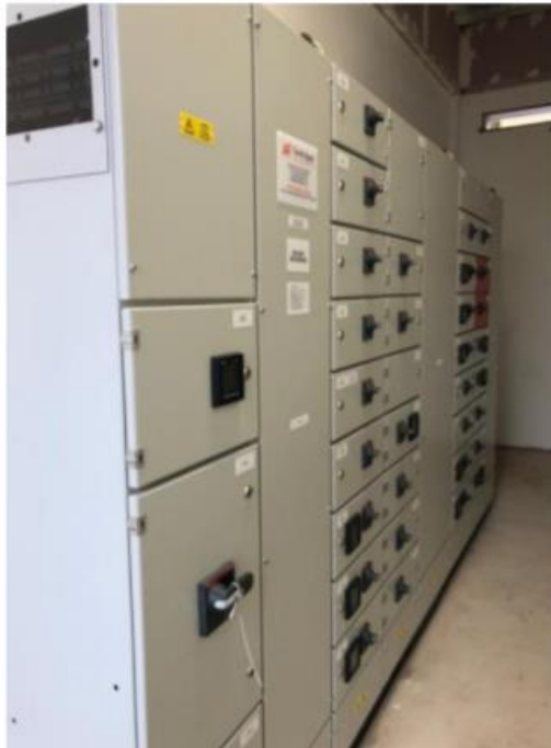
New Electric mains panel delivered and installed to the switch room
