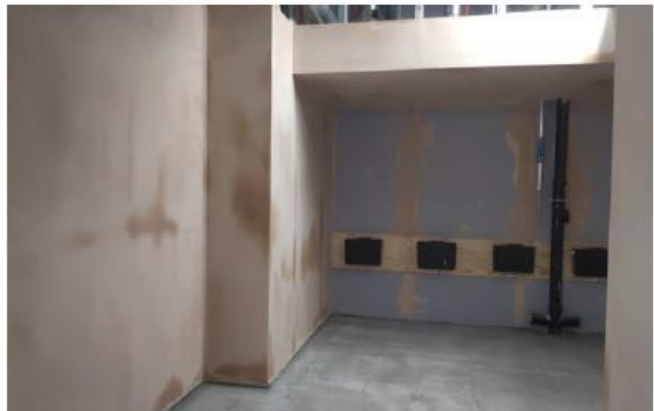
DPM to floors ready for vinyl
