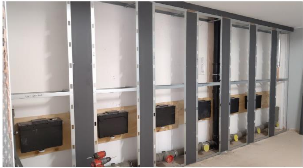
IPS to toilets ➔
