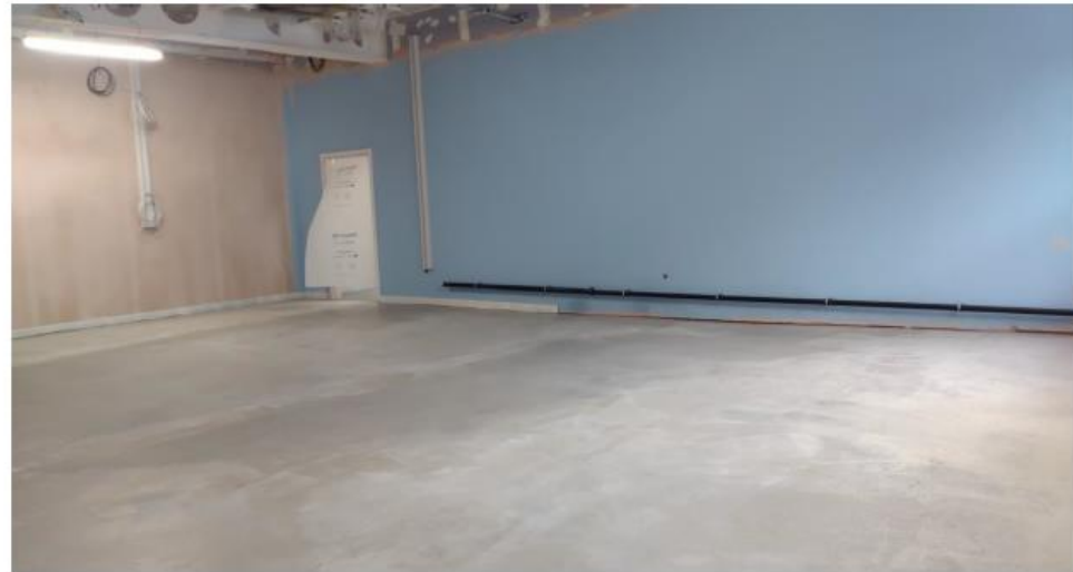
Heated rooms have allowed floor prep, dpm and latex screed to science
