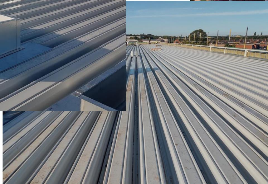
All roof decking now complete
