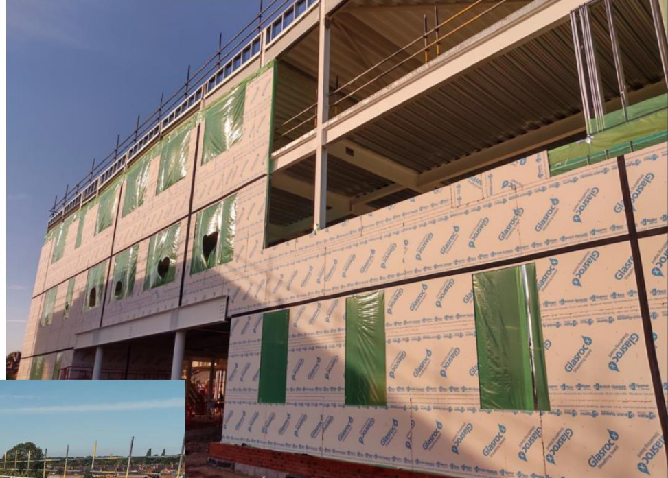
East elevation SFS complete
