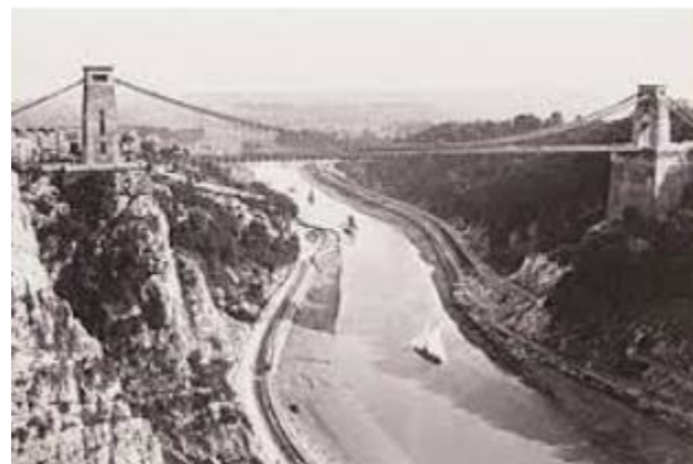
Clifton Suspension Bridge
