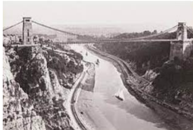
Clifton Suspension Bridge
