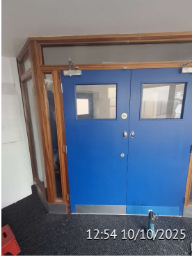
Issue 7 Left Hand Door/Change Hinges / Lift Door 10mm / Add Lipping
