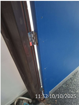
Issue 2 Right Hand Leaf Lift Up 10mm/ Change Hinges X3
