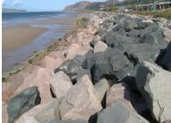
Cheap and efficient at reducing energy in waves approaching the coast.
