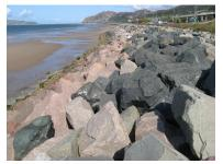
Cheap and efficient at reducing energy in waves approaching the coast.
