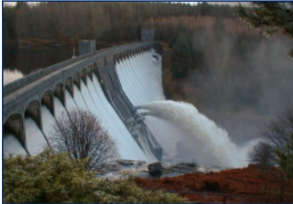
This picture shows water being released under pressure, after it has turned the turbines inside the dam to generate electricity (Laggan Dam).
