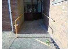
Demarcate the start/end of the ramp
