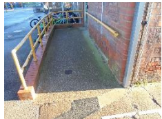
Demarcate the start/end of the ramp
