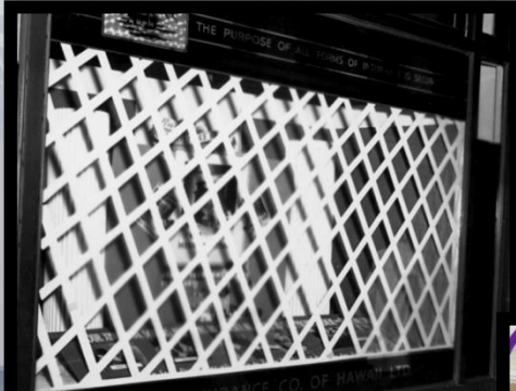
Taped window glass stops glass shattering in bomb explosion
