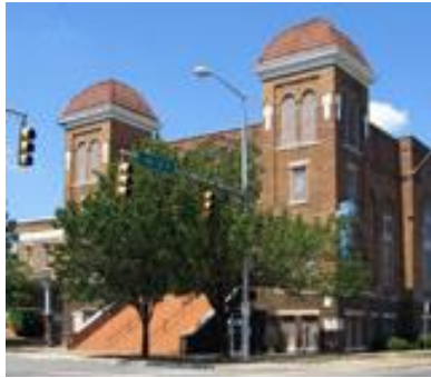
Baptist church in Alabama, USA. Most Baptist churches look like ordinary houses or town halls
