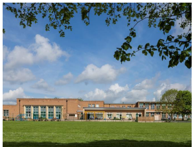
Cator Lane site
