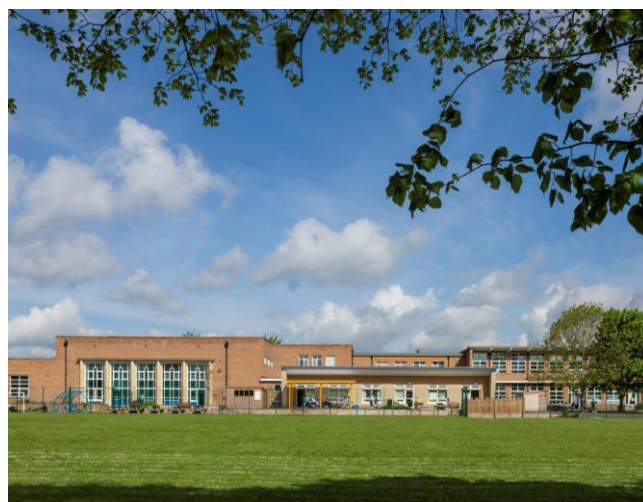
Cator Lane site
