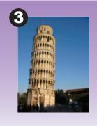
This tower is in Italy. It is actually a bell tower for the cathedral. The height of the tower is 55.86m on the low side and 56.7m on the high side. The tower has sunk on one side due to unsuitable foundations.
