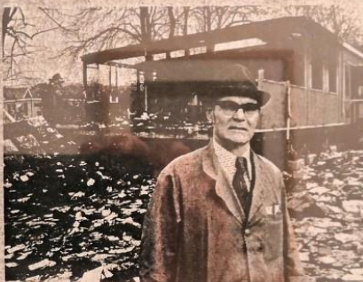
VALLEY SCHOOL'S caretaker, Mr William Blockley, in front of the burnt-out block. Police suspect arson.
