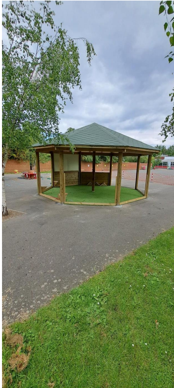
1 - The part-complete outdoor classroom. When finished it will seat up to 50 children and has a built in whiteboard.
