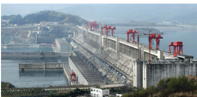
Hydroelectric dam in Hubei, China
